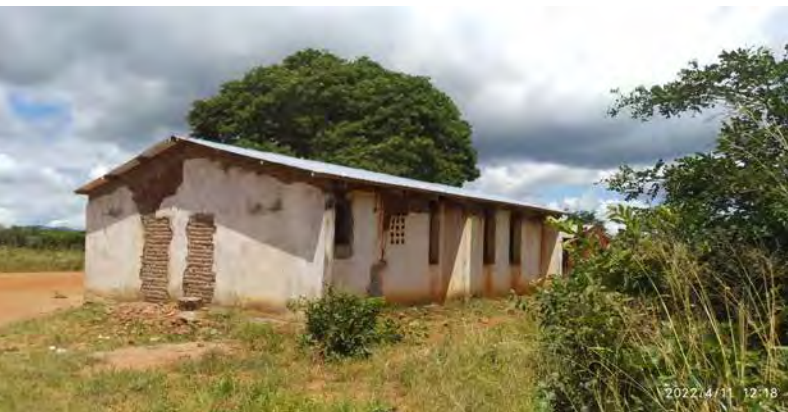
Kapilimuhoto Clinic re-roofed
