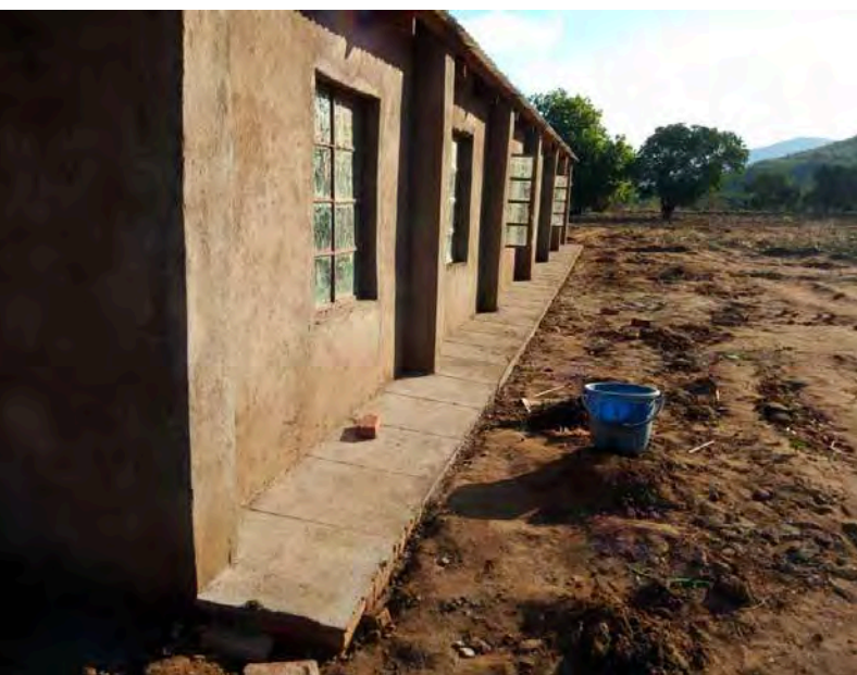
Muyegha - Vestry - finishing cement drainage
