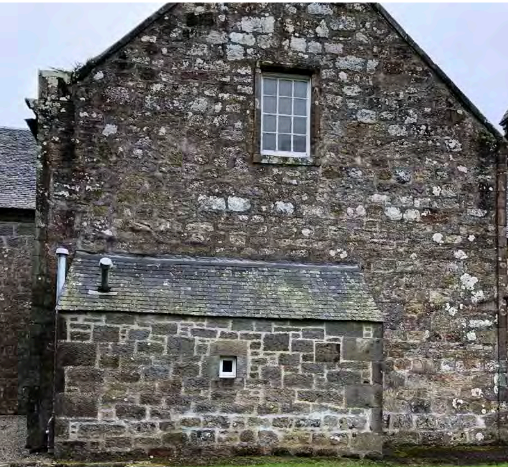
Site of new extension to replace lean-to north entrance to Church
